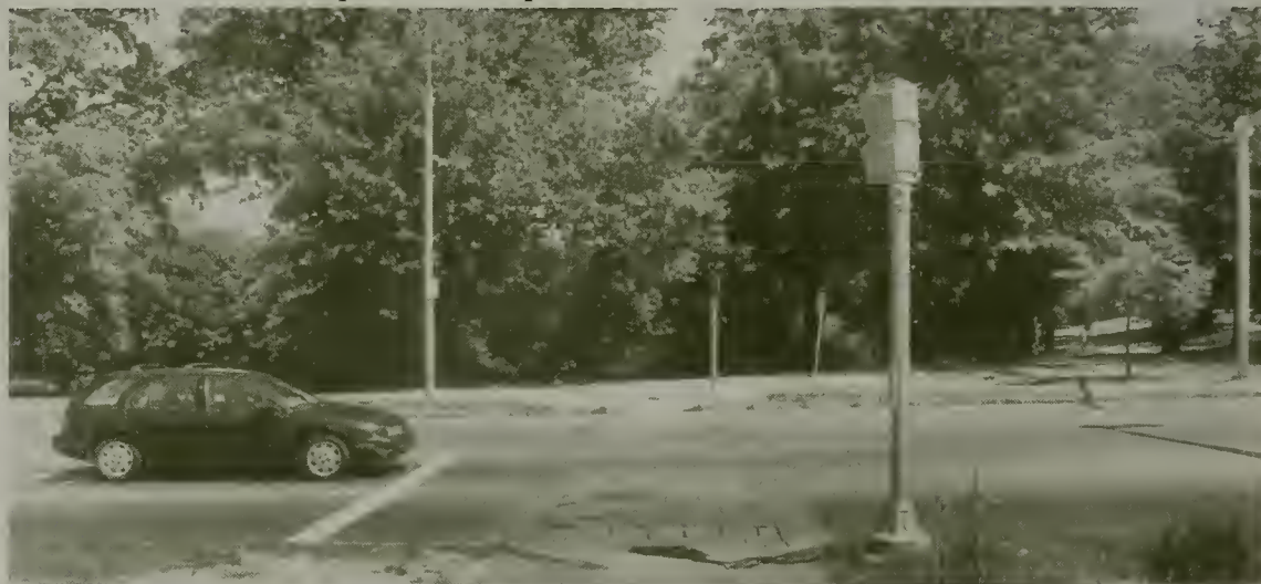
Figure 101: Back Bay Fens - Concrete walk with granite curbs and granite block crosswalk along Park Drive (Jon Crispin Photography, 1999).
