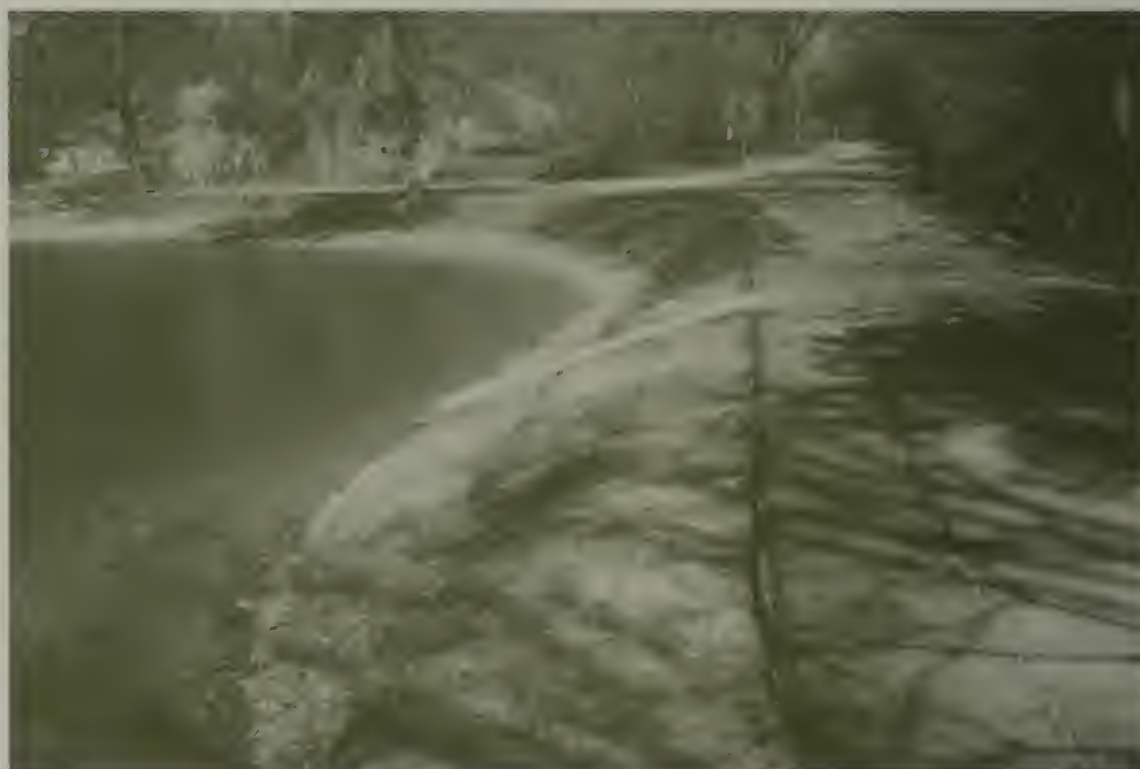
Figure 44: Jamaica Pond - Edge deteriorated by swale action at "beach" location at Perkins Street (Pressley Associates, 1998).
