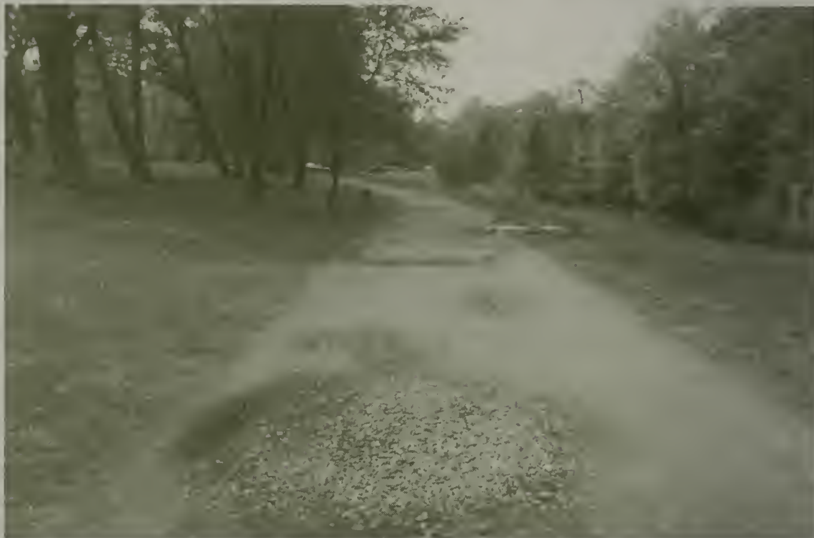
Figure 56: Riverway - Drainage and erosion along path (Pressley Associates, 1998).
