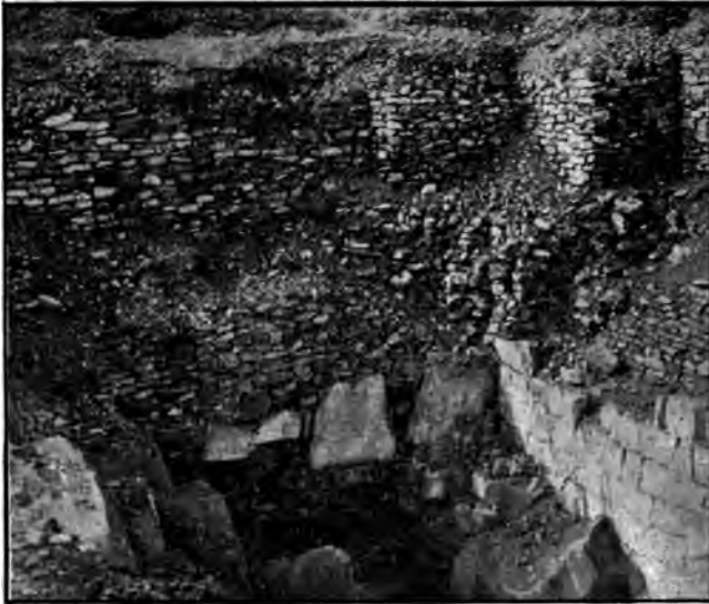
Fig. 53.—Rubble walls and chips forming the mass of the pyramid. At the right is the top of the chamber masonry.
