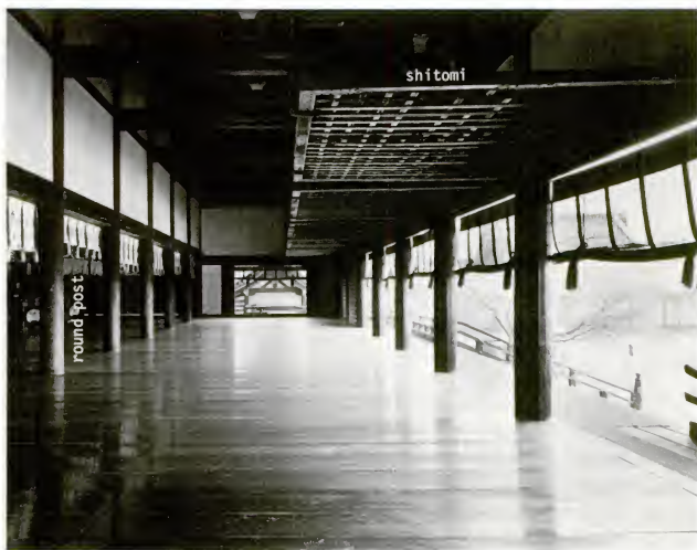
FIGURE 1. Traditional use of round posts and hinged wall panels ( shitomi ). Photograph courtesy of Shokokusha, Tokyo.
